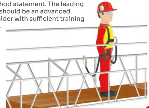
Figure 11: Construction of Prefabricated Beams and temporary boarding
