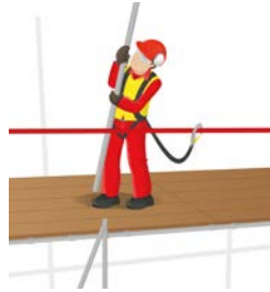
Figure 5: Hemping behind collective fall protection
